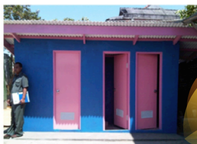
Setelah direnovasi / After renovated
